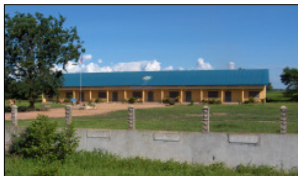
Figure 6: Primary school in Cambodia
