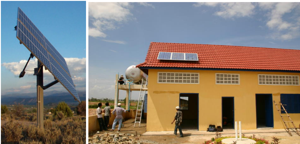
▲ Left: Solar panels on a tracker system can lead to an increase in performance up to 40%. Right: A static established solar panel system
