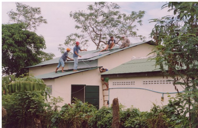
▲ Installation of solar panels at an orphanage in Cambodia
